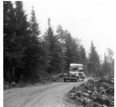
The Gunflint Trail under construction Photo courtesy of the Fink family
